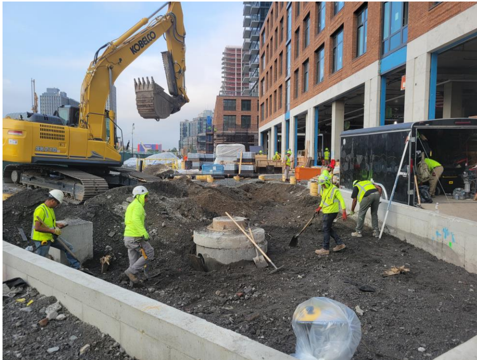
Photo 1: G&M excavating in the northeastern part of Society Brooklyn within the SPW (facing south)
