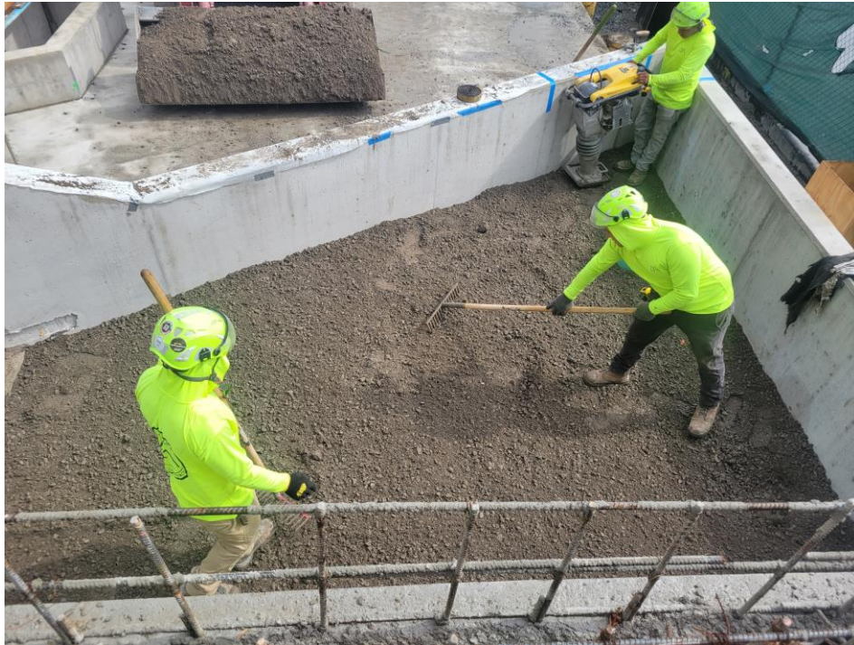
Photo 1: G&M backfilling with NYSDEC-approved fill in the southeastern part of Sackett Place within the SPW (facing north)
