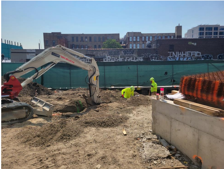
Photo 1: G&M excavating in the eastern part of the SPW in Sackett Place (facing east)
