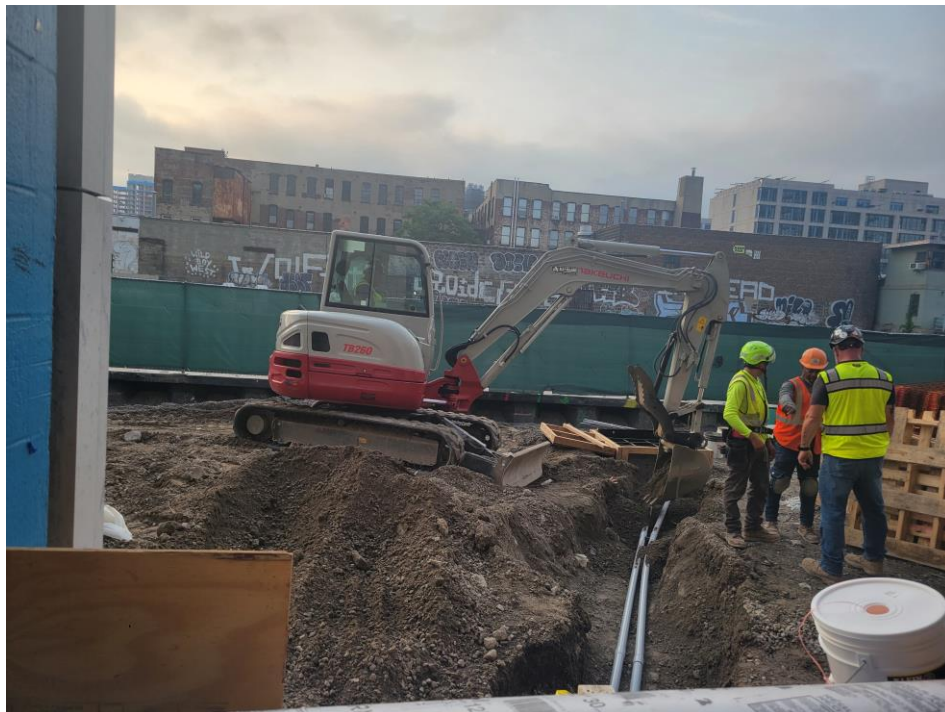
Photo 2: G&M excavating for utility installation in the central part of the SPW in Sackett Place (facing east)
