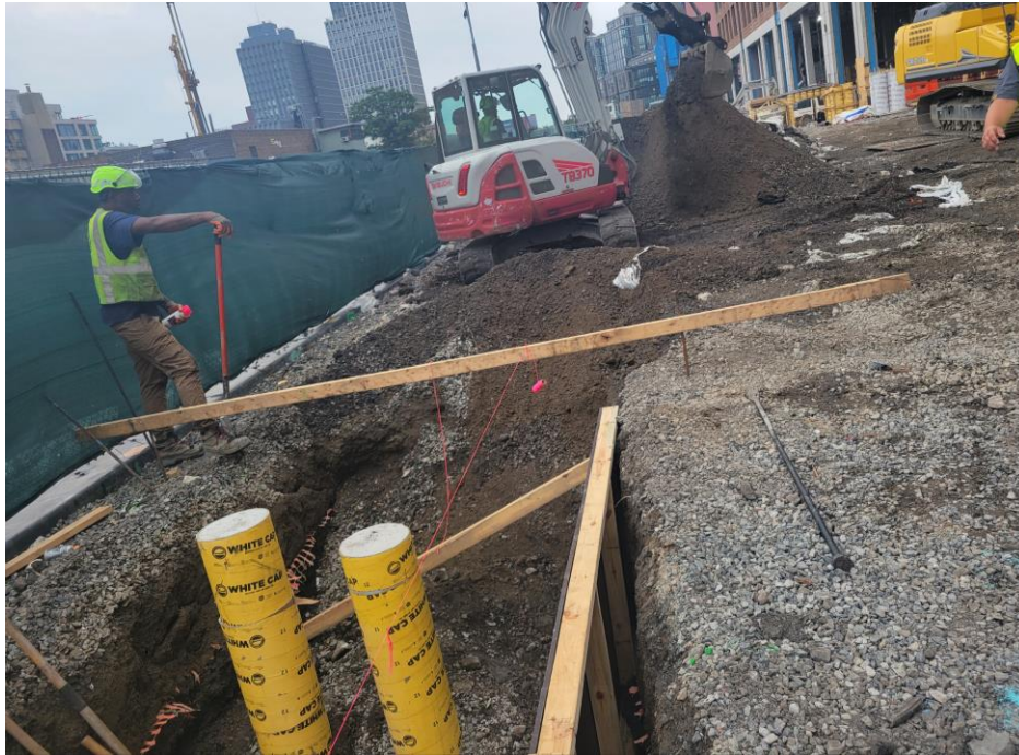
Photo 1: G&M excavating for foundation element installation in the eastern part of the SPW in Society Brooklyn (facing south)
