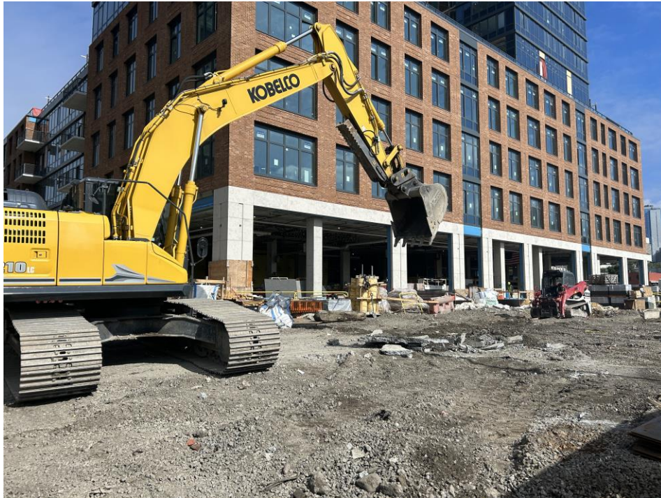
Photo 1: G&M demolishing a concrete slab in the northern part of the SPW (facing northwest)
