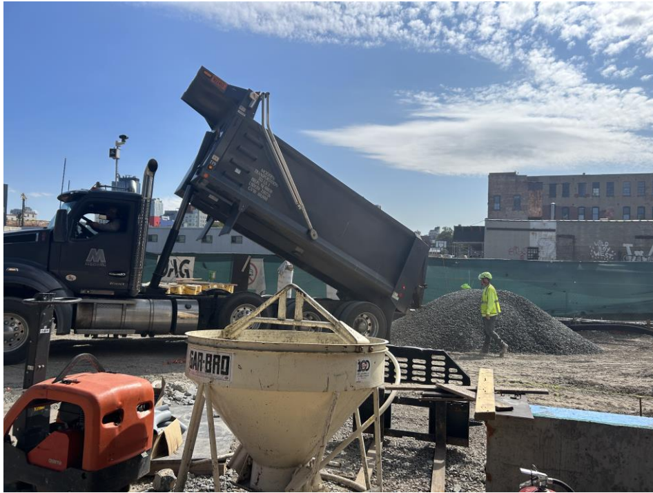
Photo 1: G&M importing a truckload of 0.75-inch stone (facing east)
