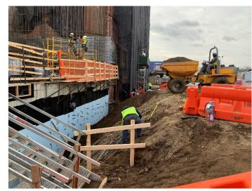
Photo 2 – Looking north, Structure Tech loads trucks with soil and concrete debris from SP3 for offsite disposal to Fairless Landfill.
