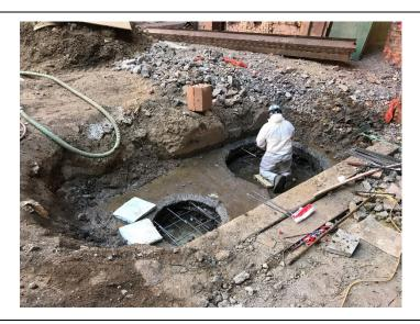
Photo 2 – Facing south, StructureTech New York pours the structural concrete cap at TH-SUMP-5 and TH-SUMP-5-Auxiliary.
