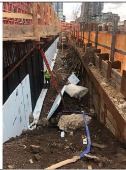
Photo 2 – Looking northwest, Structure Tech begins backfilling the north side of the boiler house superstructure after waterproofing and insulation work are complete.
