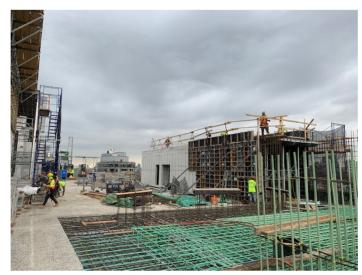
Photo 3 – Facing south, StructureTech New York Inc. continues construction of the turbine hall foundation.
