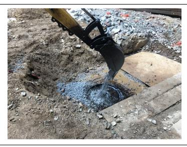
Photo 2 – Looking north, Brookside Environmental pours the 2 ft thick concrete plug at TH-SUMP-1.
