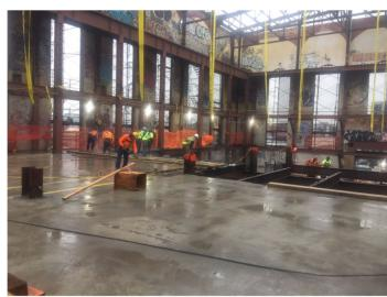
Photo 3 – Looking northeast, Structure Tech pours concrete for one of the boiler house superstructure decks.
