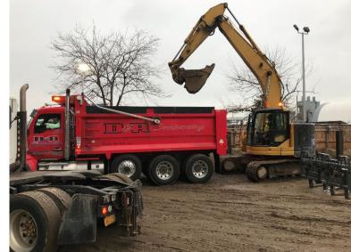
Photo 2 – Looking east in the west yard. Structure Tech loads trucks with soil from the north property line soil stockpile for offsite disposal.
