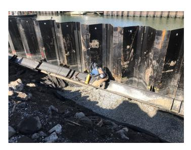
Photo 3 – Facing northeast, Land and Sea Construction Corp. drills, installs, and grouts the tieback at the bulkhead.
