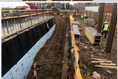
Photo 3 – Looking northwest, Structure Tech begins compacting the backfill soil along the north side of the boiler house superstructure.
