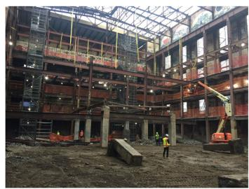
Photo 3 – Looking northeast, Structure Tech pours concrete for the upper decks of the boiler house superstructure.
