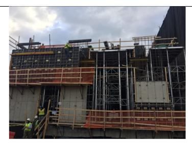
Photo 2 – Looking north, Structure Tech prepares for slab pour on the third floor of the boiler house superstructure.
