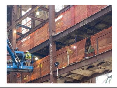
Photo 2 – Looking south, Structure tech continues construction of the boiler house superstructure.
