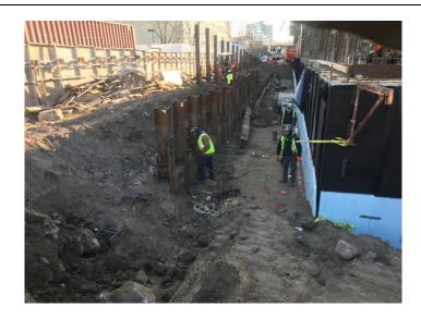
Photo 2 – Looking southeast, Structure Tech continues backfilling the north side of the boiler house superstructure after waterproofing and insulation work are complete.
