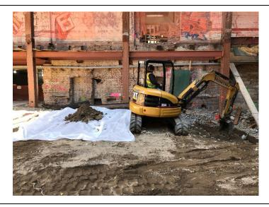
Photo 2 – Looking east, Brookside Environmental pumps oily water displaced during the turbine hall sump remediation process to totes for future offsite disposal.
