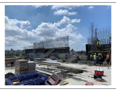
Photo 2 – Facing southeast, Maspeth Welding continues steel installation/restoration in the turbine hall.
