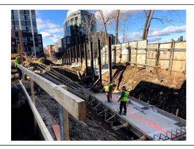
Photo 2 – Facing southeast, Nordest Services LLC demolishes existing features in the northeast portion of the site.
