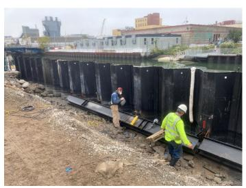
Photo 3 – Facing northwest, Land and Sea Construction Corp. continues installing tiebacks for the bulkhead.
