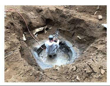
Photo 3 – Facing east, StructureTech New York pours the structural concrete cap at TH-SUMP-4.
