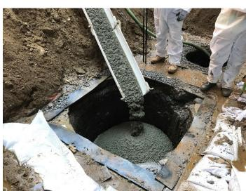
Photo 3 – Facing west, view of TH-SUMP-2 after the concrete plug pour was completed.
