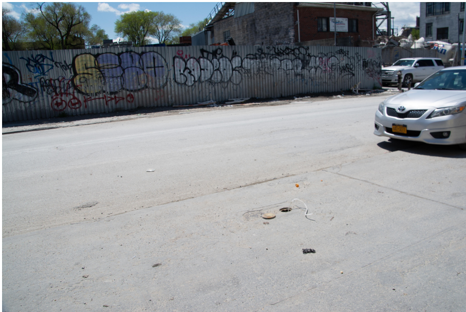
SG-9 Opened for Inspection; Boerum Street
