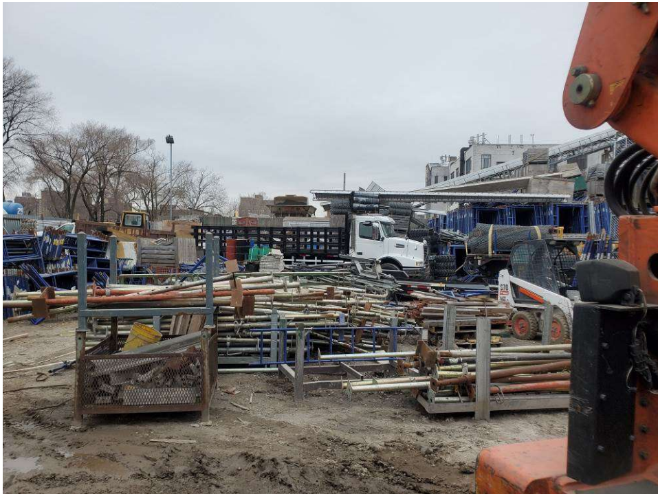
Activity near MW-10; MW-11, MW-12, and SG-8 in background
