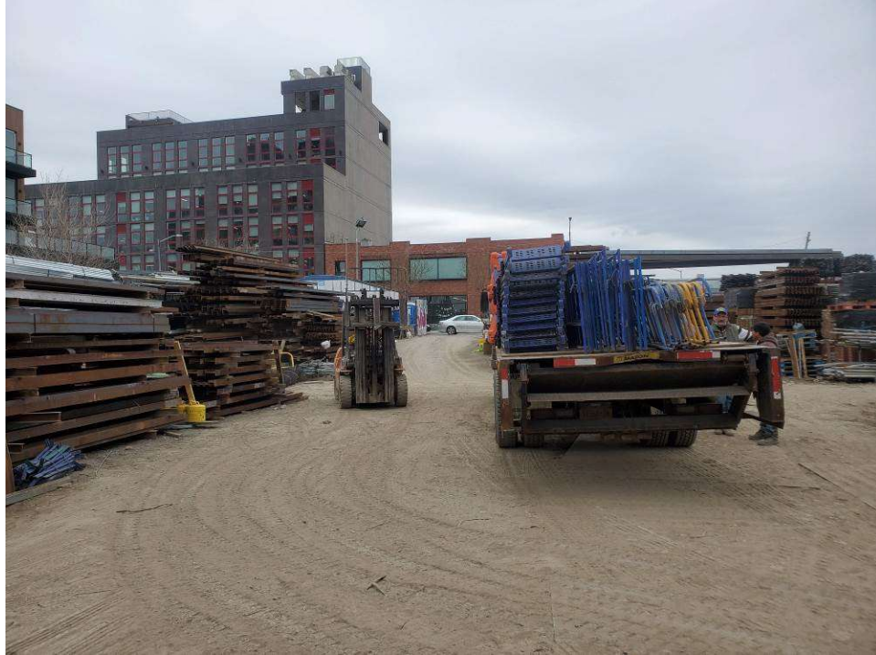
Activity in yard near MW-10; looking toward Boerum Street
