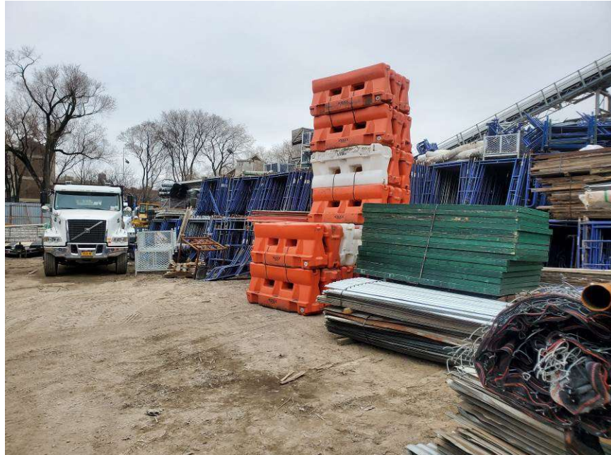
Activity near MW-11, MW-12, and SG-8; cement plant in background
