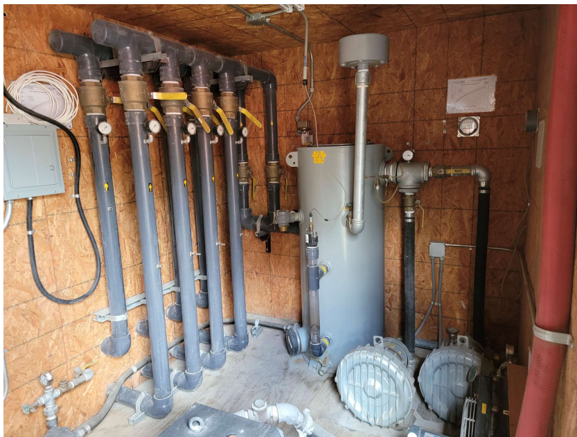
SVE Line 1B: front pipe to right; position of frozen valve shown
