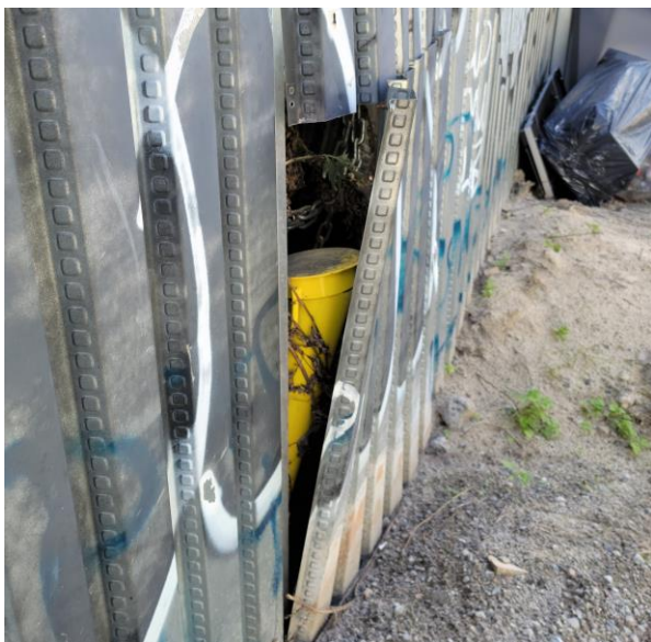
SG-5R behind vapor probe gate
