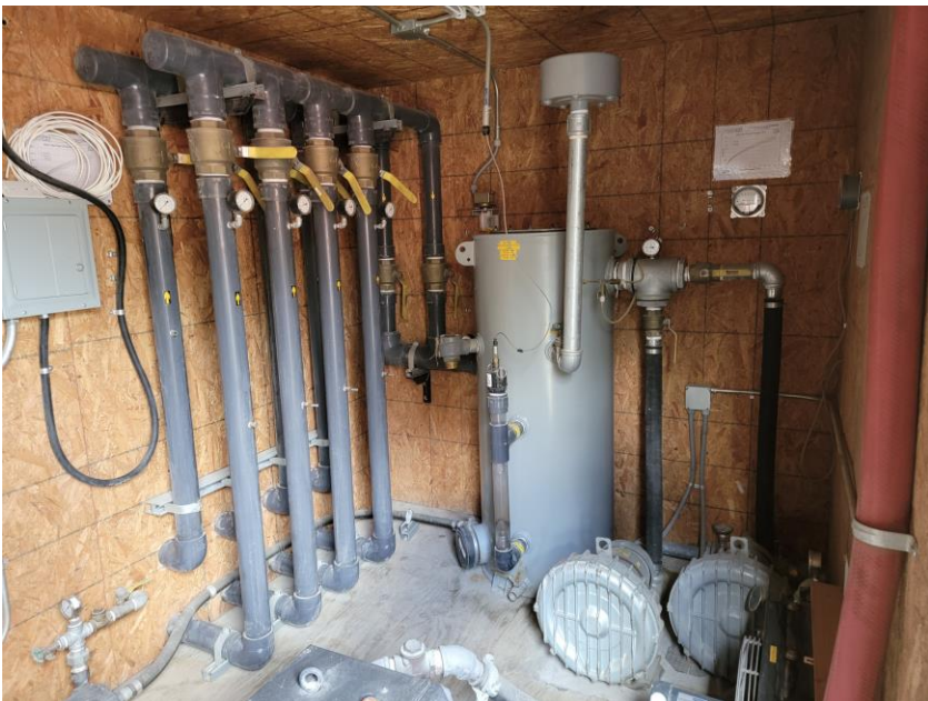
SVE Lines 1 through 3 open
