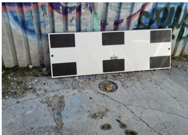
MW-7 needing cover replacement and cleaning
