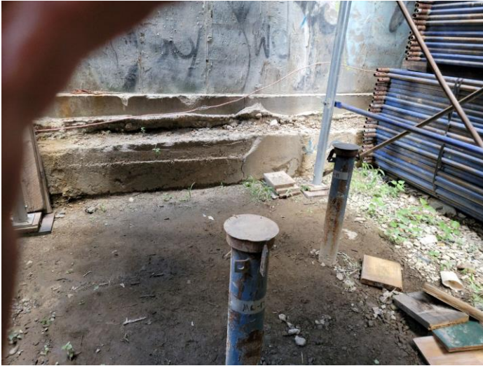
Monitoring Wells 7 and 8
