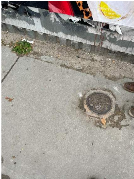
DESCRIPTION: Flush Mount Well in Sidewalk
