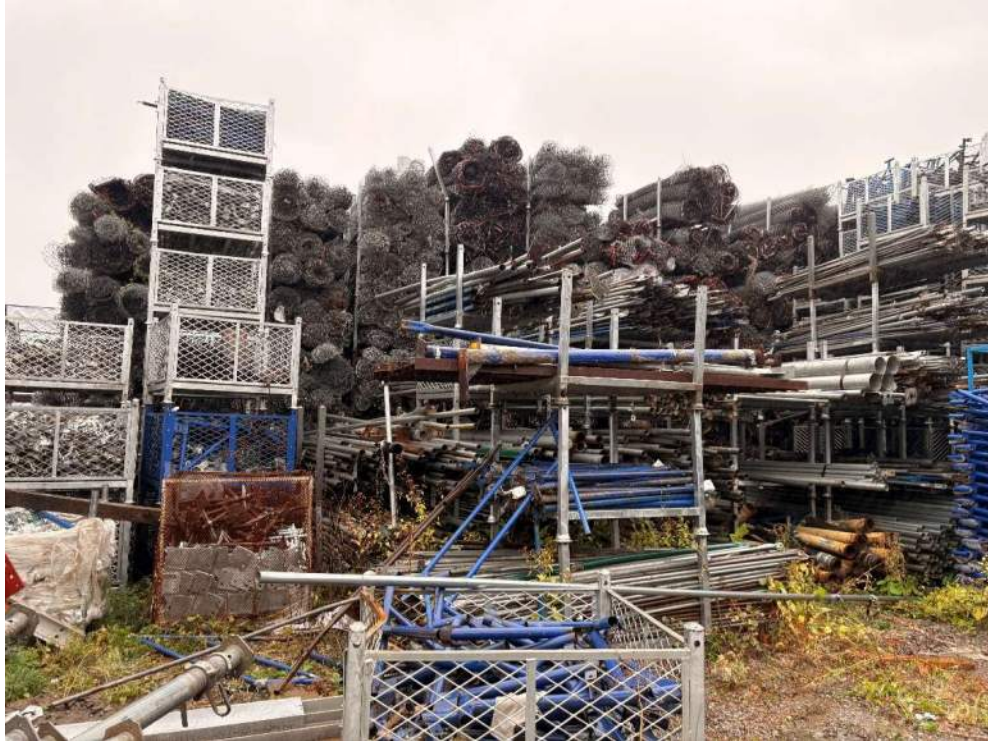
Description: Scaffolding on Site
