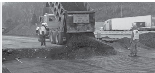
Image 7 End dumping aggregate fill on top of Tensar TriAx Geogrid over soft subgrade.
