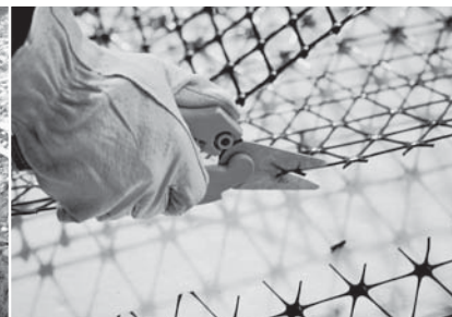
Image 5 Cutting Tensar TriAx Geogrid is easily achieved.
