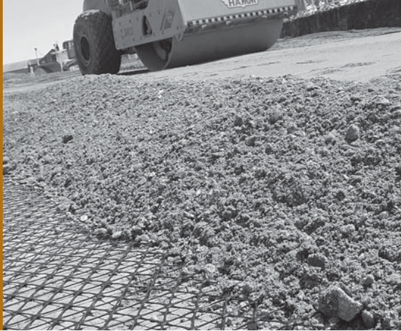
Image 10 Compacting the aggregate fill.
