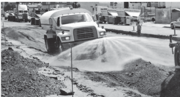
Image 9 Moistening the fill before compaction.
