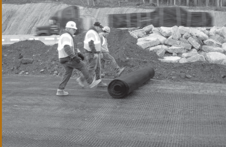
Image 2 Rolling out Tensar® TriAx® Geogrid.
