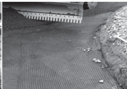
Image 4 Placing Tensar TriAx Geogrid to accommodate curves.
