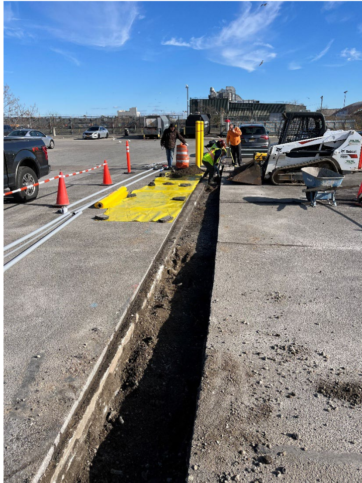
Photo 1 Excavation Looking West to East
