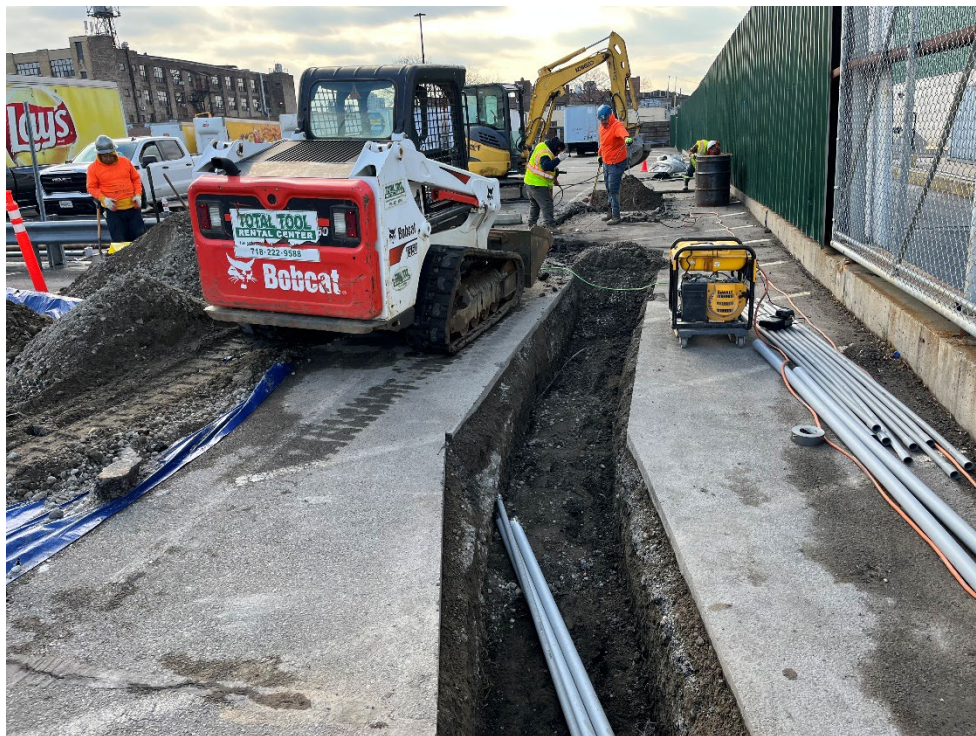
Photo 2 Excavation Looking East to West
