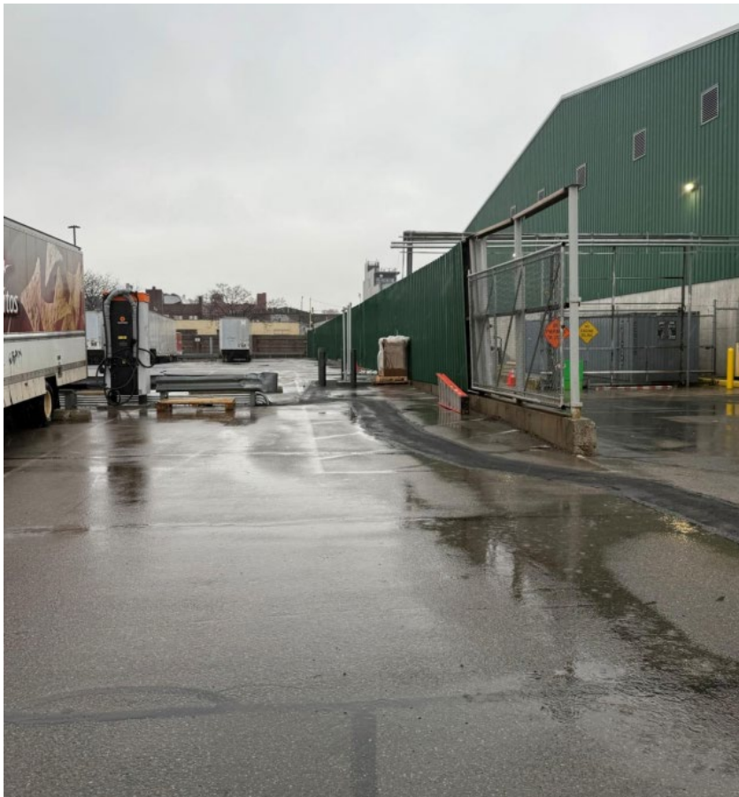
Photo 6 Repaved and Restored Pavement
