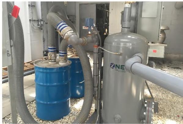
Photo 5: SVE inlet and moisture separator
