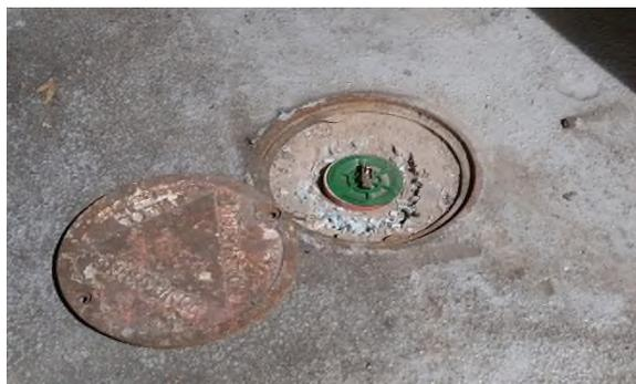
Photo 7: Groundwater monitoring well
