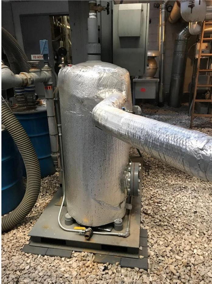
Photo 5: SVE inlet piping to knockout tank
