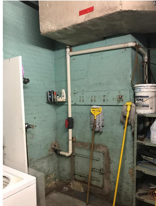
Photo 10: SJHS SSDS piping in boiler room and extraction point R2
