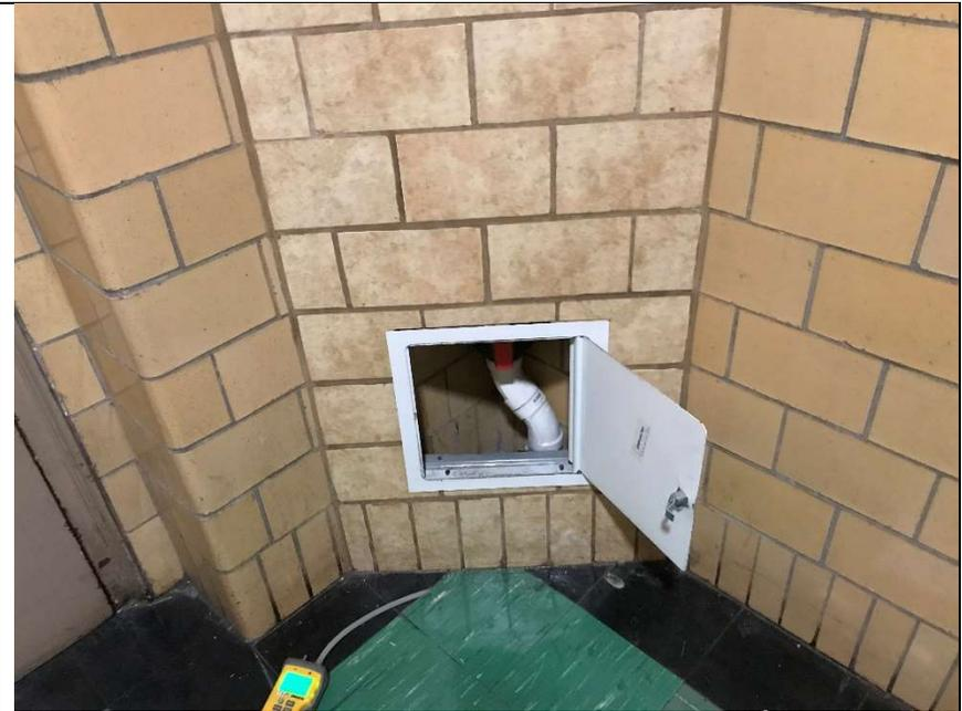
Photo 12: SJHS SSDS piping and monitoring point R12 location
