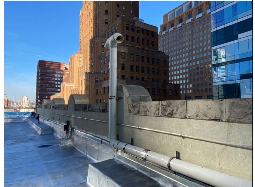
Photo 14: SJHS SSDS piping and exhaust
