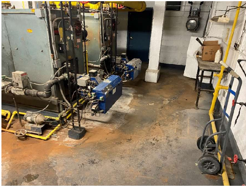
Photo 11: 80 Willoughby basement slab boiler room
