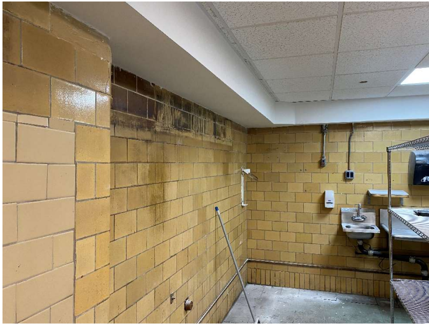
Photo 13: Former kitchen hood (BPS) location at 80 Willoughby.
