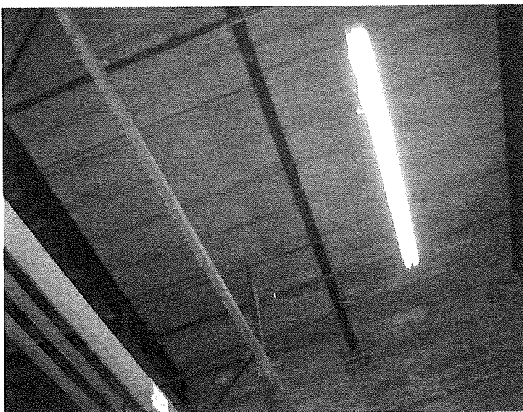
CONCRETE CEILING IN WAREHOUSE AREA
