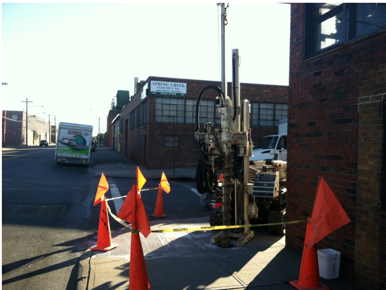
Monitoring well installation
