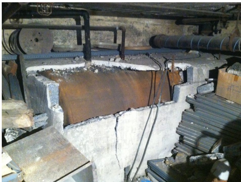
Fuel Oil Tank in concrete vault in basement
