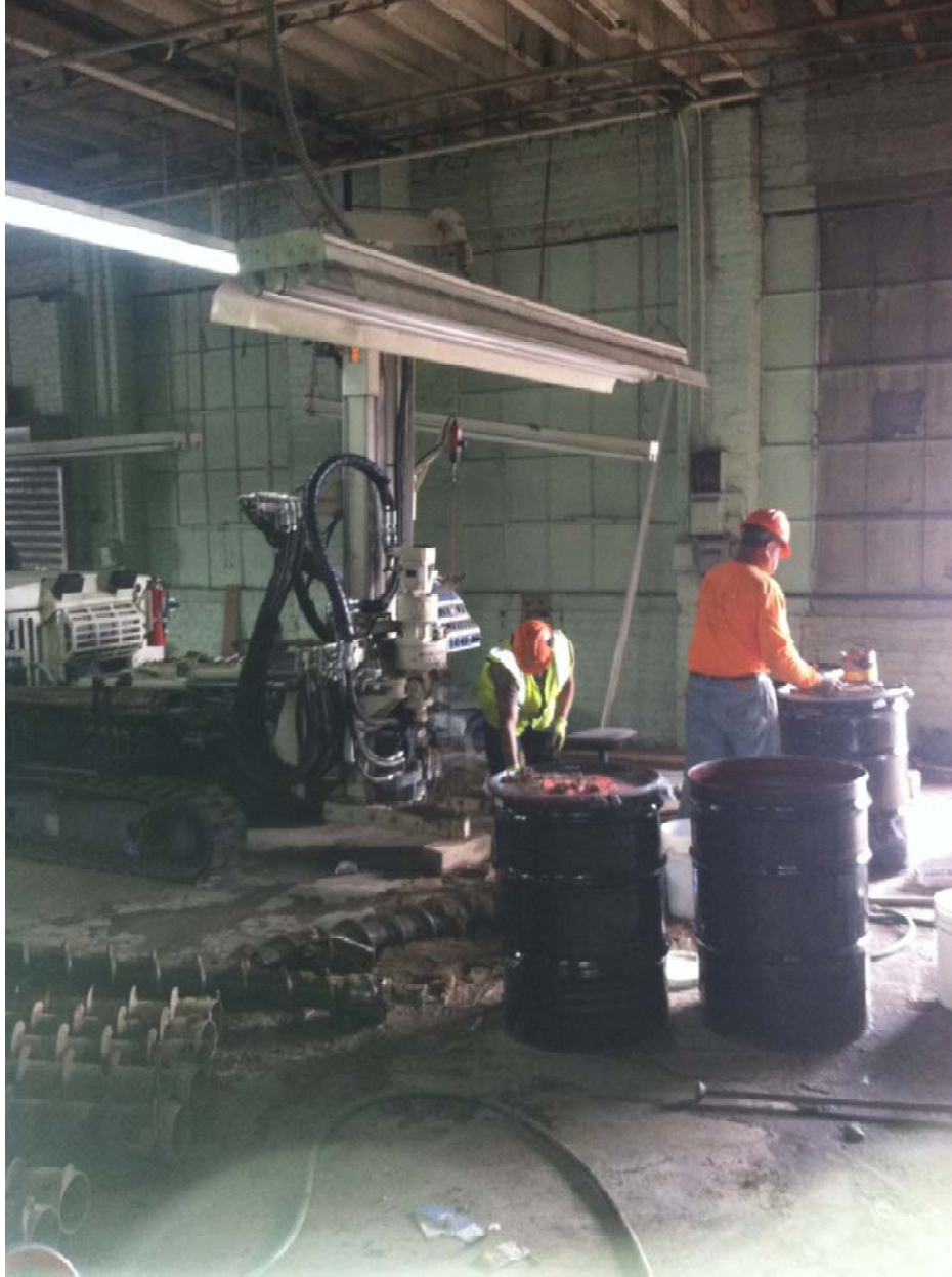
Drilling equipment and drums for investigation-derived waste
