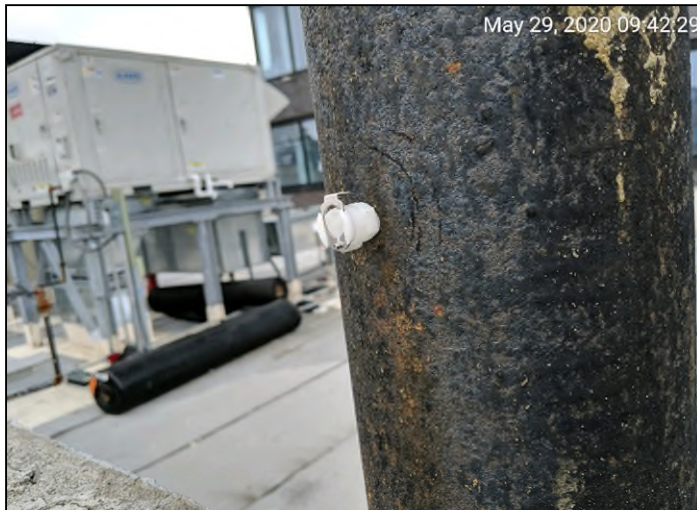
Photograph 5: Sub-slab venting system exhaust stack with newly installed sample port.
