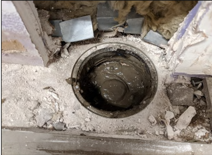
Photograph 5: Sub-slab vacuum monitoring MP-1 following decommissioning with concrete.
