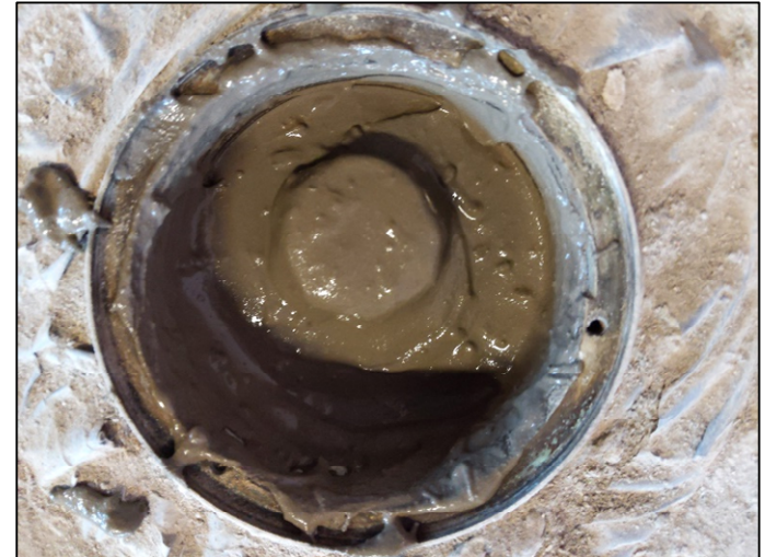
Photograph 6: Sub-slab vacuum monitoring MP-3 following decommissioning with concrete.
