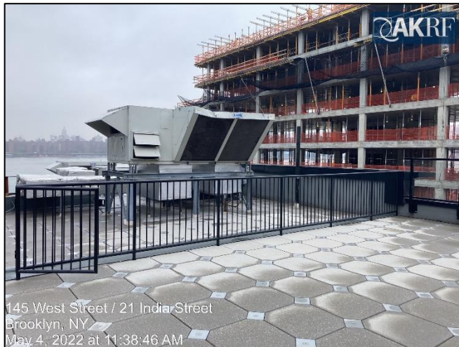
Photograph 7: Sub-slab venting system exhaust stack; view facing northwest.
