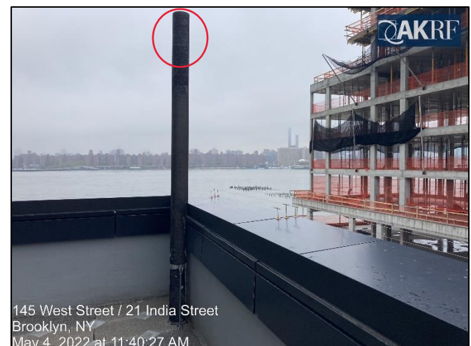
Photograph 8: Exhaust stack sample port.
