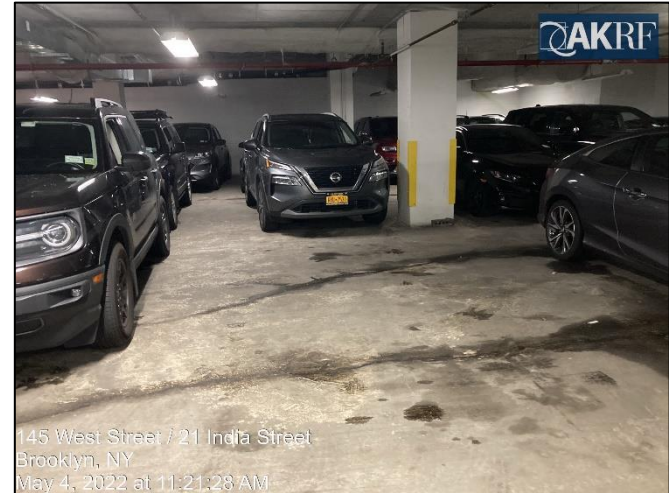
Photograph 10: Surficial cracks observed in Building B floor slab.
