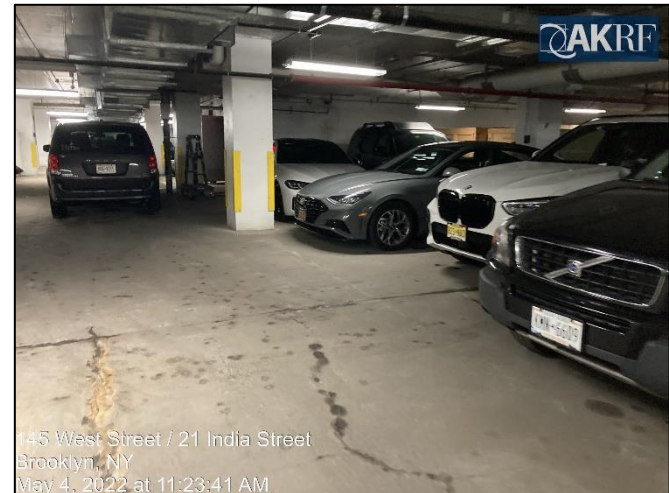
Photograph 12: Sealed surficial cracks in Building B floor slab.
