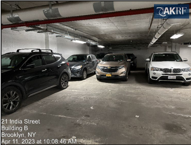
Photograph 9: Building B below-grade parking garage.
