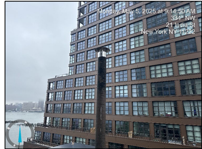
Photograph 2: Installed rain cap on fourth-floor exhaust riser pipe; view facing northwest.
