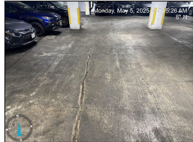
Photograph 6: Sealed surficial cracks observed in Building B floor slab.
