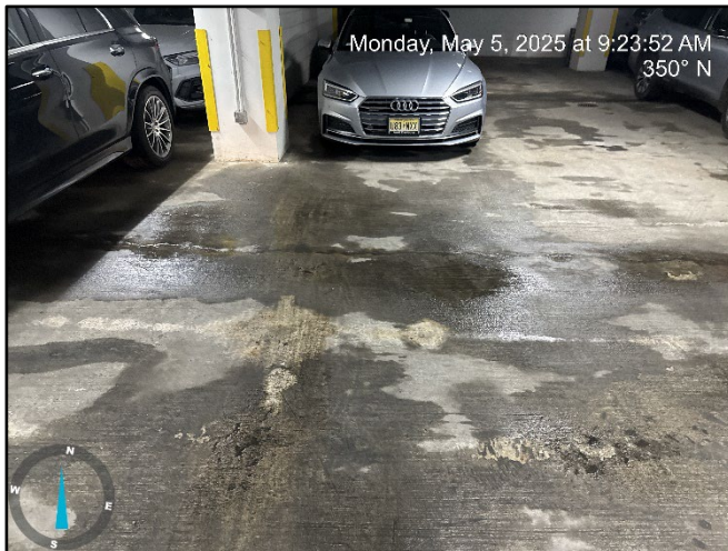
Photograph 3: Building B below-grade parking garage.
