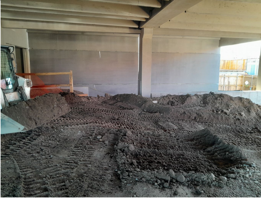
Photo 3: Facing East Southeast; Soiled being graded in area B3 in preparation for foundation work.
