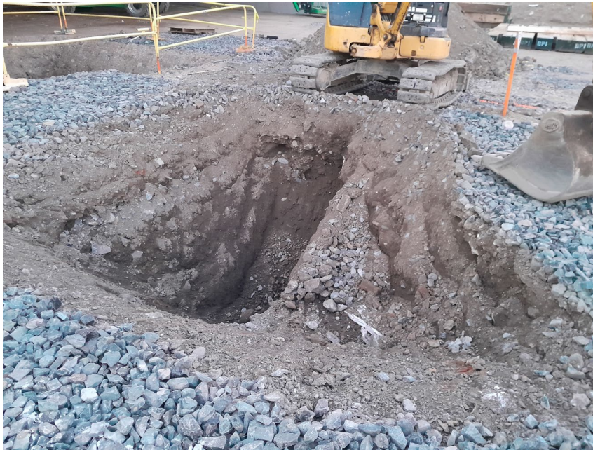
Photo 1: Facing South; Kingdom starting excavation in B2 to expose pile cap in preparation to install prefabricated concrete columns.
