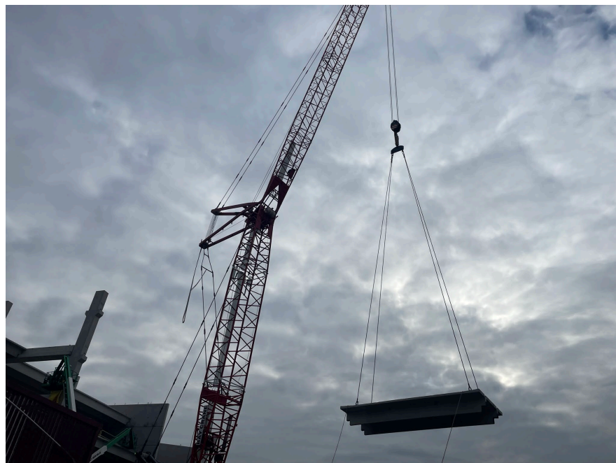
Photo 2: Facing Southwest; Concrete form being added to the superstructure.
