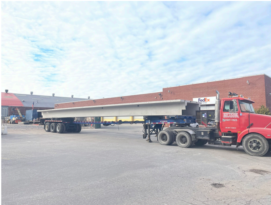
Photo 1: Facing Southwest; prefabricated concrete form being delivered to site.
