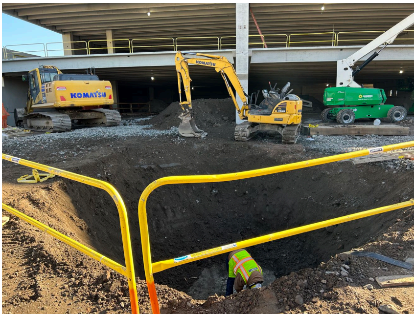
Photo 2: Facing east; excavation to uncover previously poured pile cap to assist future precast erection.
