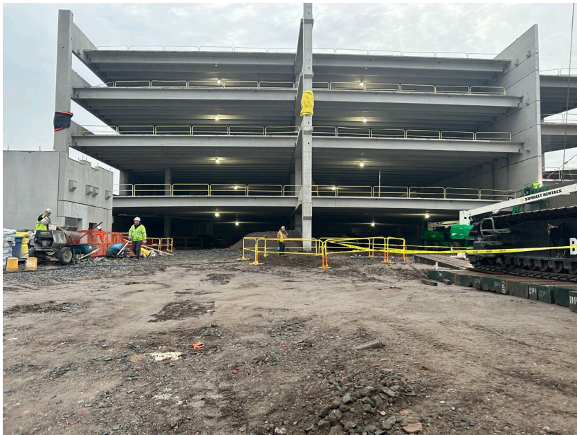
Photo 2: Facing east; status of area excavated to previously poured pile cap to assist future precast erection.
