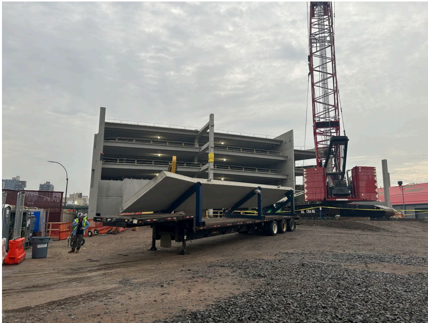
Photo 1: Facing southeast; delivery of prefabricated concrete forms to site.
