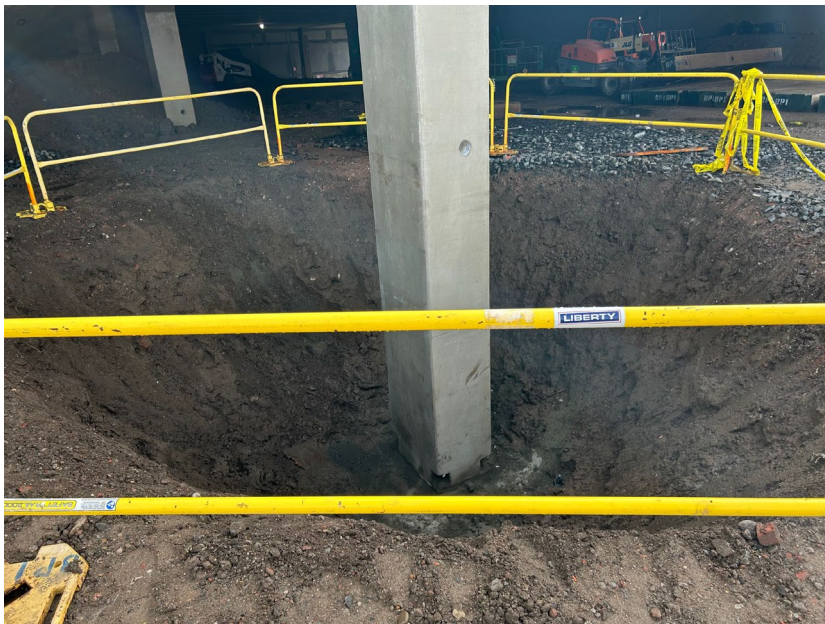
Photo 2: Precast vertical column was erected in the area of the previously exposed pile cap in grid A2.
