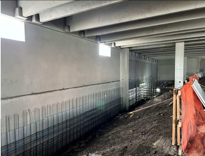
Photo 2: Facing east, rebar placement for retaining wall in grid A2.
