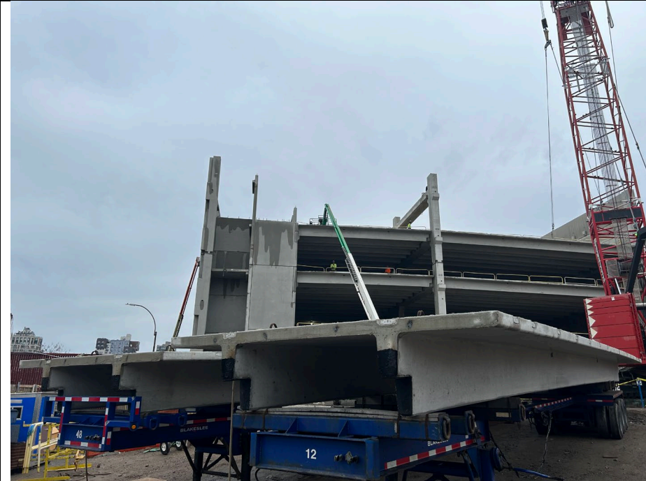
Photo 3: Looking southeast, preform concrete delivery and progress of superstructure.
