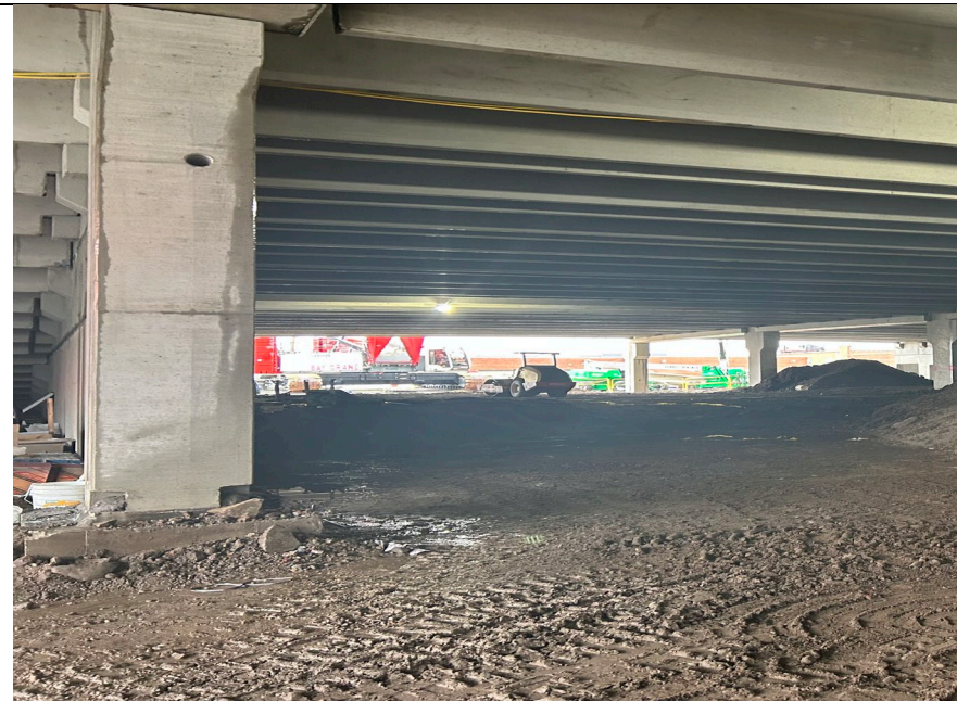
Photo 2: Facing north, general site conditions under superstructure.
