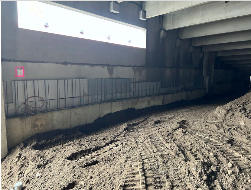
Photo 2: Facing west, previously poured wall in grid B3 with forms removed and soil previously displaced for retaining wall was backfilled around it.
