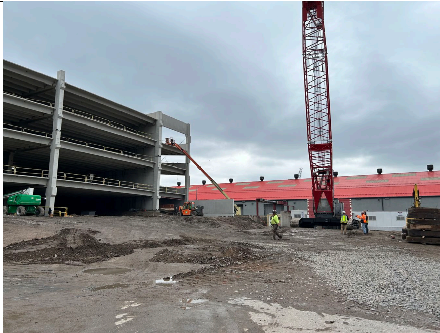
Photo 3: Looking southeast, progress of superstructure and crane in final position to accommodate excavation of piling foundation.
