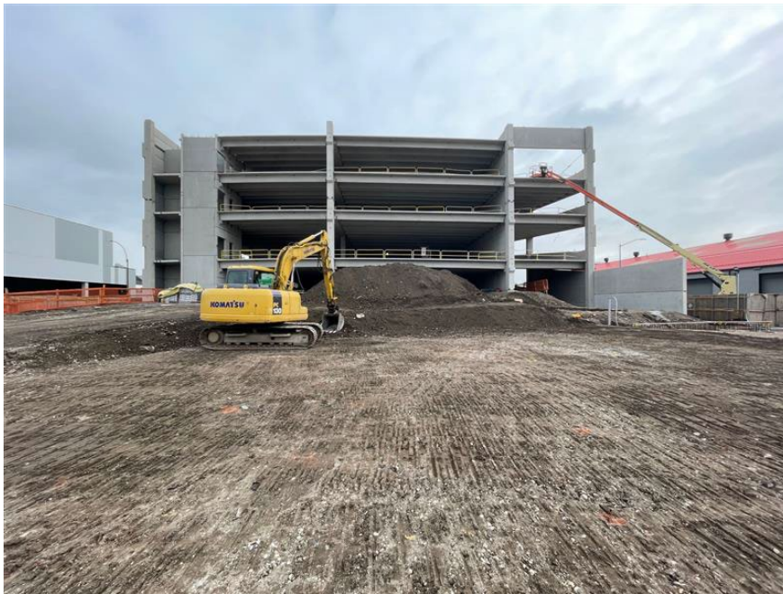
Photo 4: Grading status at the end of the day.
