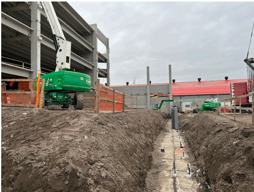
Photo 4: Progress of uncovered foundation elements and newly placed concrete preforms at the end of the day.
