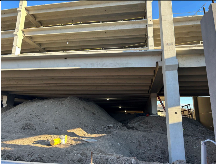
Photo 3: Looking southeast, excavated material stockpiled under superstructure. Material will be graded in place.
