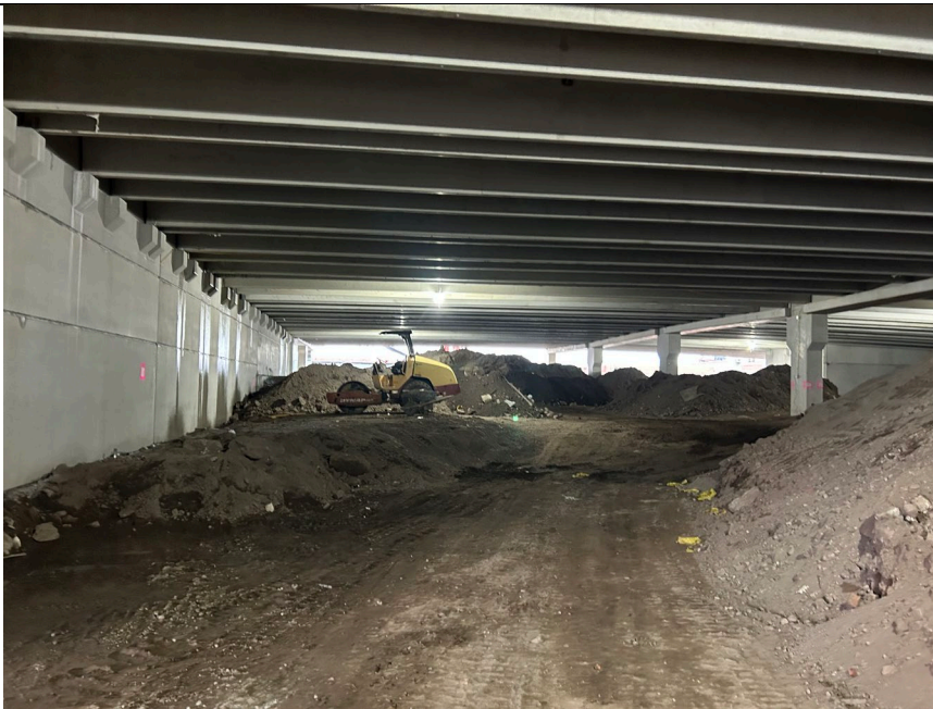
Photo 2: Facing north, grading and material stockpiling under the superstructure.
