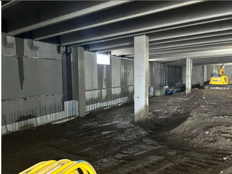
Photo 3: Looking southeast, grading around the previously poured concrete in grids A2 and A3.
