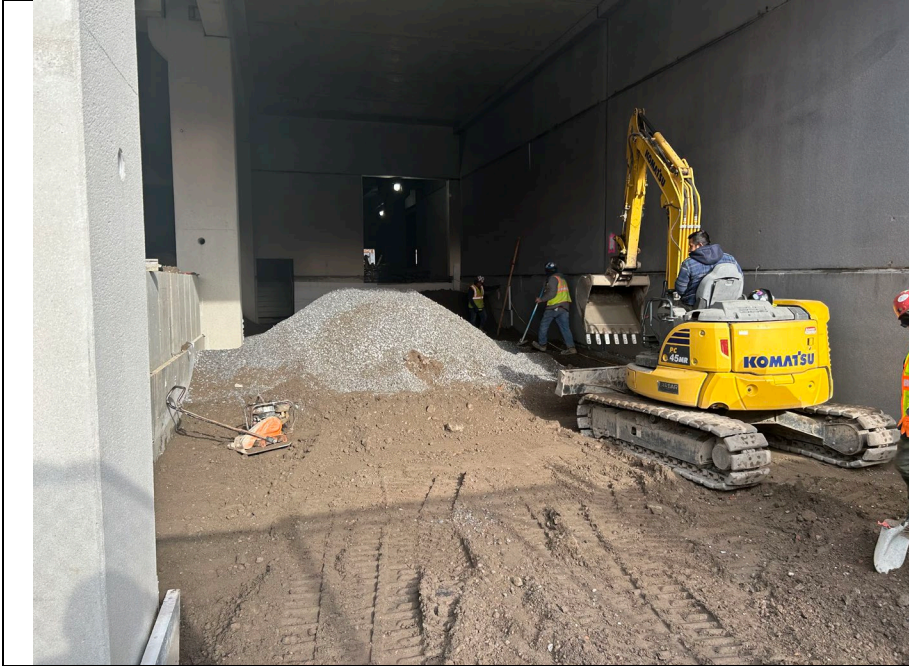
Photo 3: Progress of stone delivery and grading along south side of grid B3.
