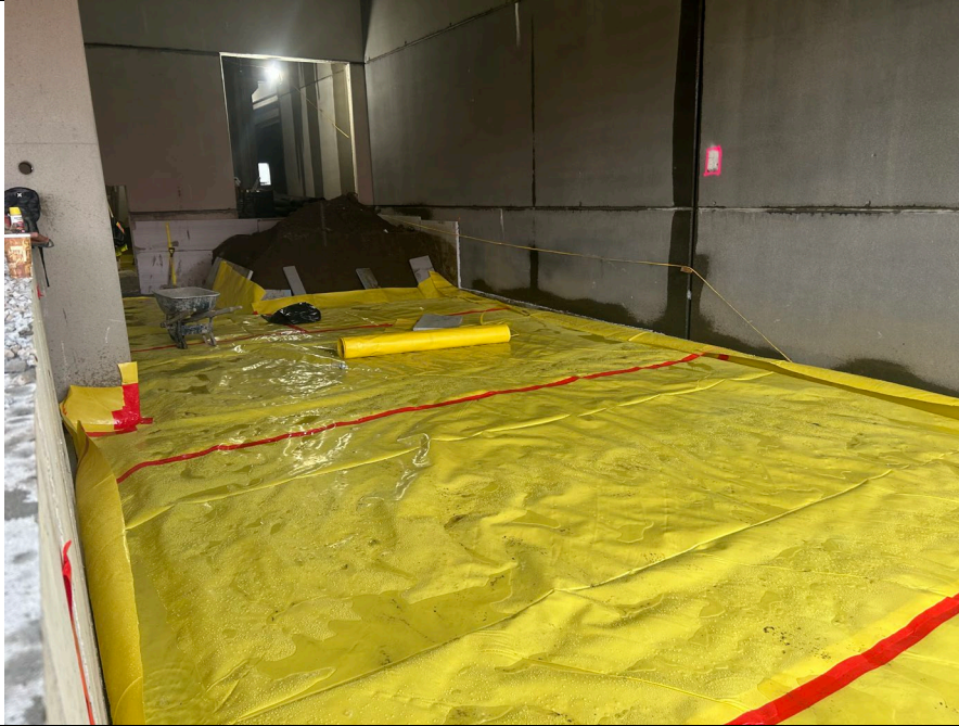
Photo 3: Progress of vapor barrier installation along south side of grid B3. Endlaps were taped in accordance with manufacturer's specs.
