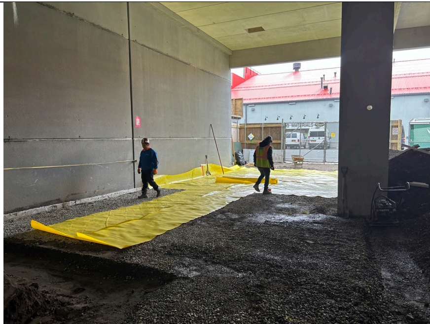
Photo 2: Facing east, beginning of vapor barrier installation in grid B3.
