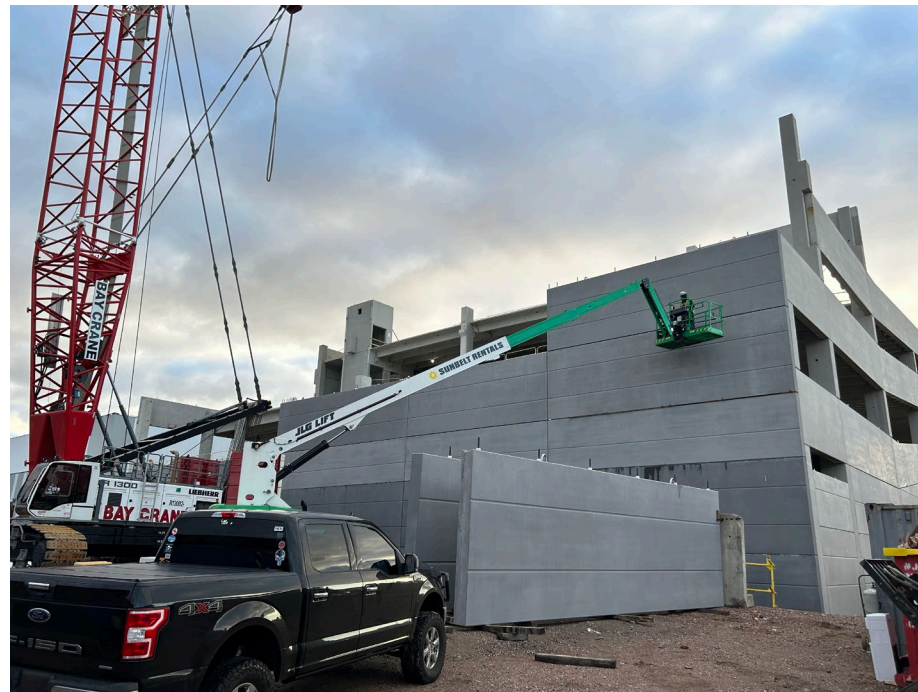
Photo 1: Facing south, superstructure status at beginning of day.
