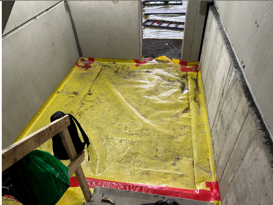
Photo 3: Progress of vapor barrier installation along south side of grid B3. Image shows completed installation in stairwell.
