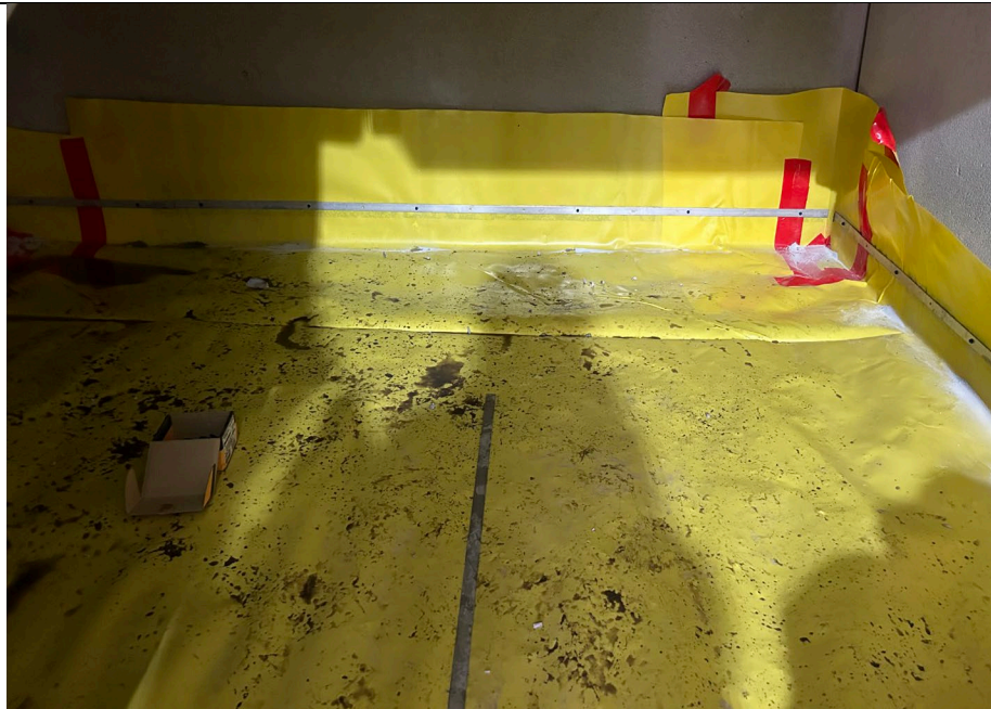
Photo 2: Detail of vertical vapor barrier installation against precast wall; applying double-sided tape prior to securing the vapor barrier to the tape with a termination bar in grid B3.
