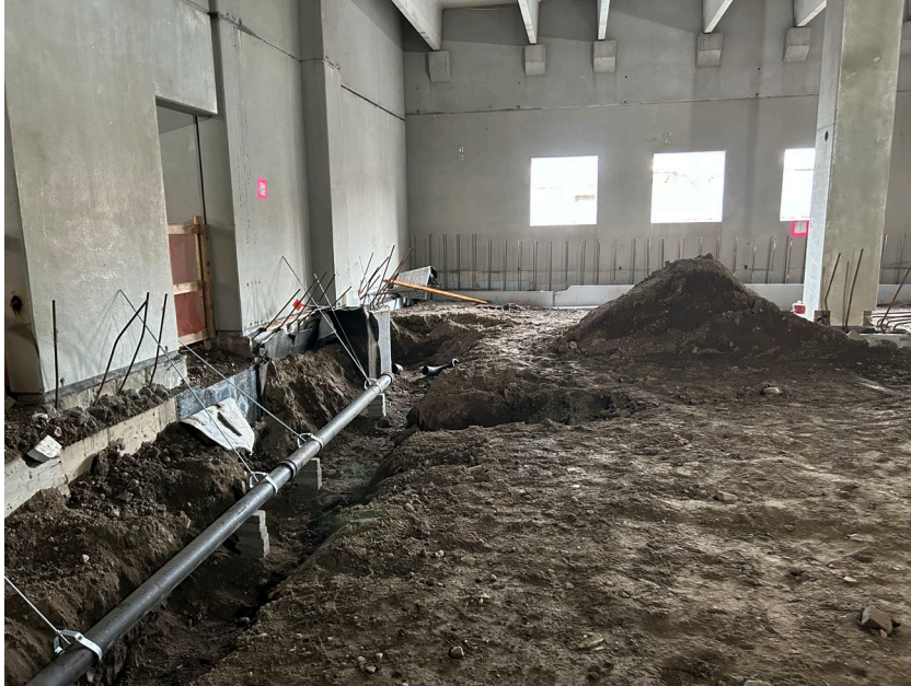
Photo 4: Facing east in grid A3, progress of utilities installation.
