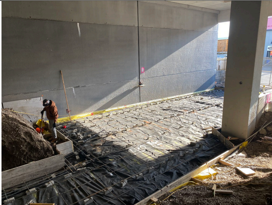
Photo 3: Progress of rebar installation ahead of concrete pouring in grid B3.
