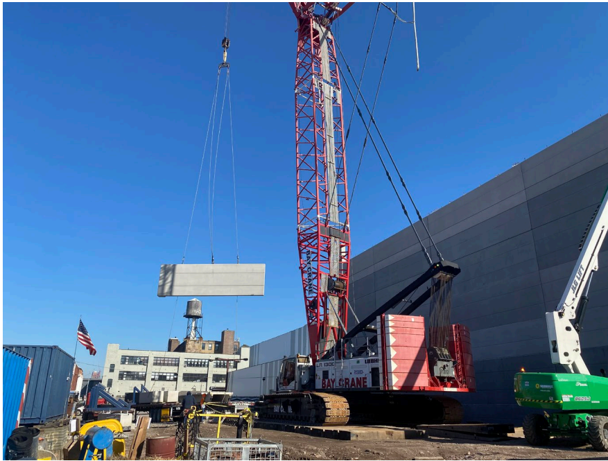
Photo 1: Facing east, concrete prefabricated pieces being placed on superstructure.
