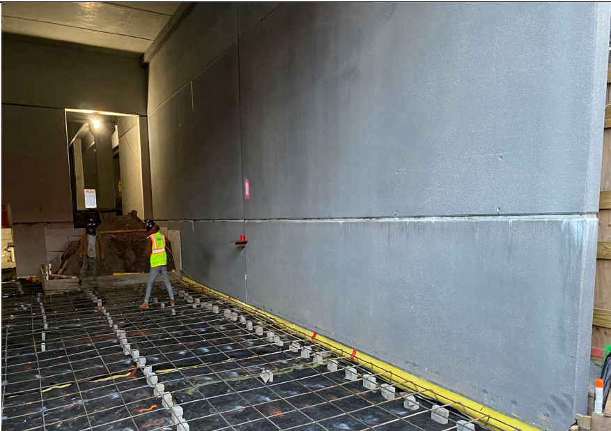
Photo 2: Facing east, rebar and forms installed to prepare for concrete pour.
