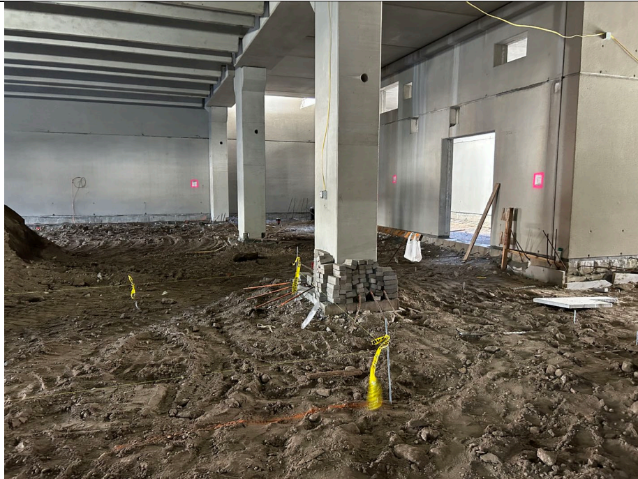
Photo 3: Utilities installation completed in grid A3 and trenches were backfilled.
