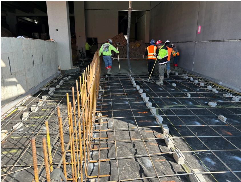
Photo 1: Concrete pouring begins in grid B3.
