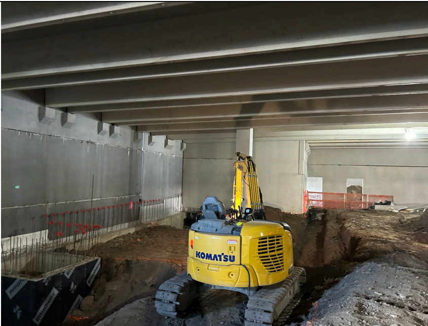
Photo 2: Trenching for utilities installation in grids A2 and A3.
