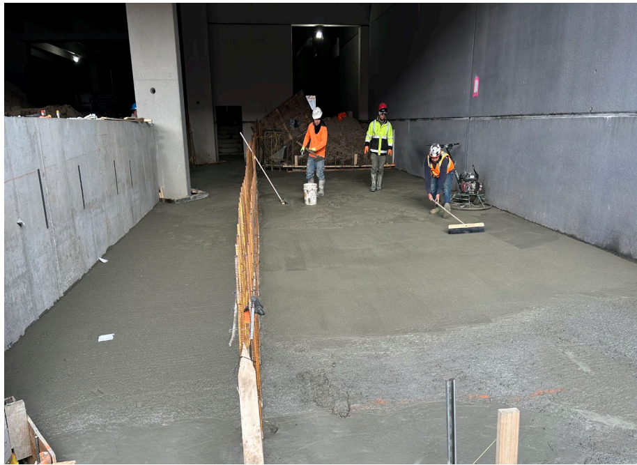
Photo 4: Concrete being leveled after pouring in grid B3.
