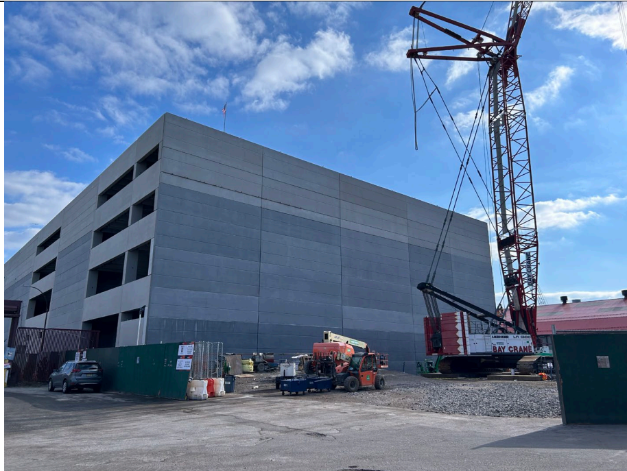
Photo 3: Facing southeast; final status of superstructure at the end of the day as Blakeslee finished concrete erection.
