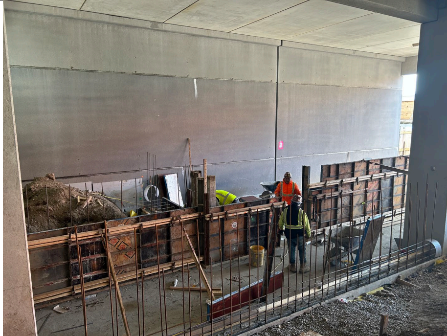
Photo 3: Concrete forms and rebar placement in grid B3.
