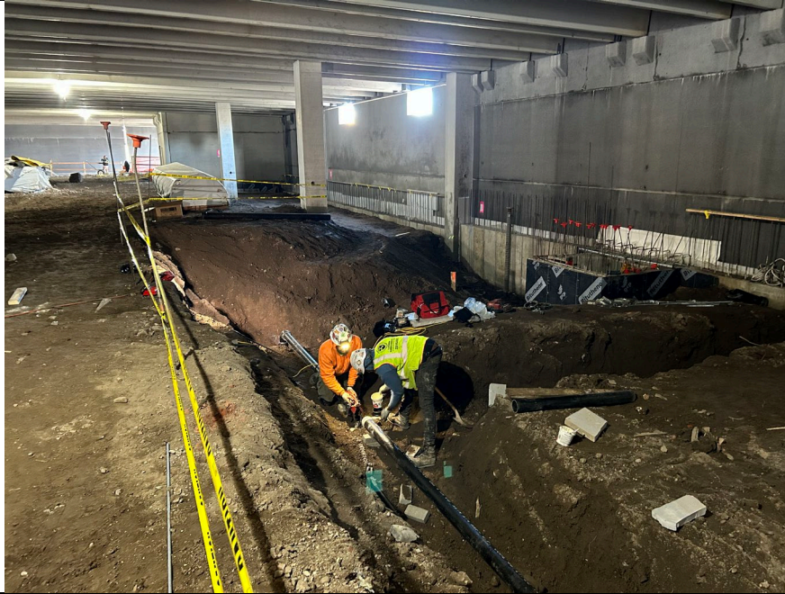
Photo 3: Plumbing installation in grids A2 and A3.
