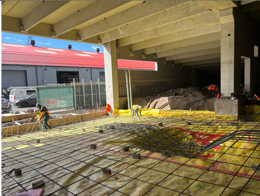
Photo 3: Progress of vapor barrier installation by Kingdom in grid B3.
