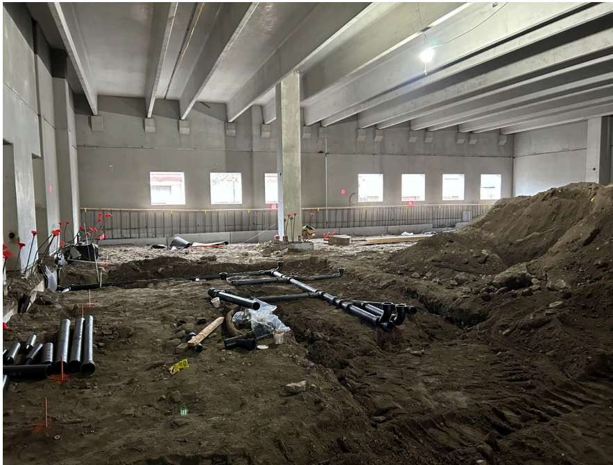
Photo 1: Status of completed plumbing in grid A4 office space. Areas will be backfilled after sign-off obtained. No soil movement today.
