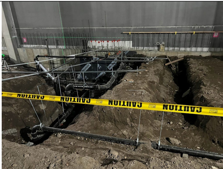
Photo 2: Status of the plumbing installation in the north end of grids A2 and A3.
