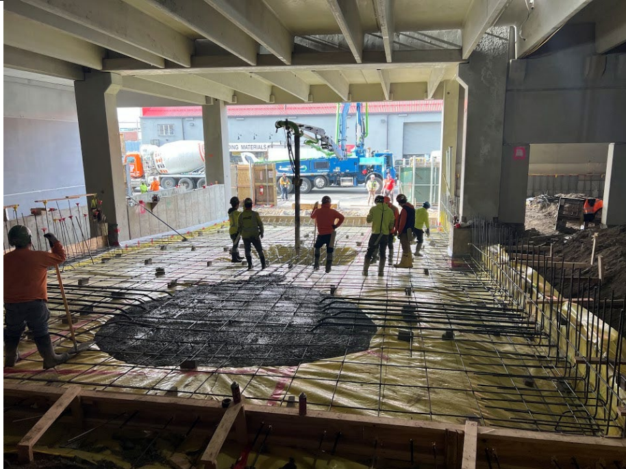
Photo 3: Progress of concrete pouring by Kingdom in grid B3.
